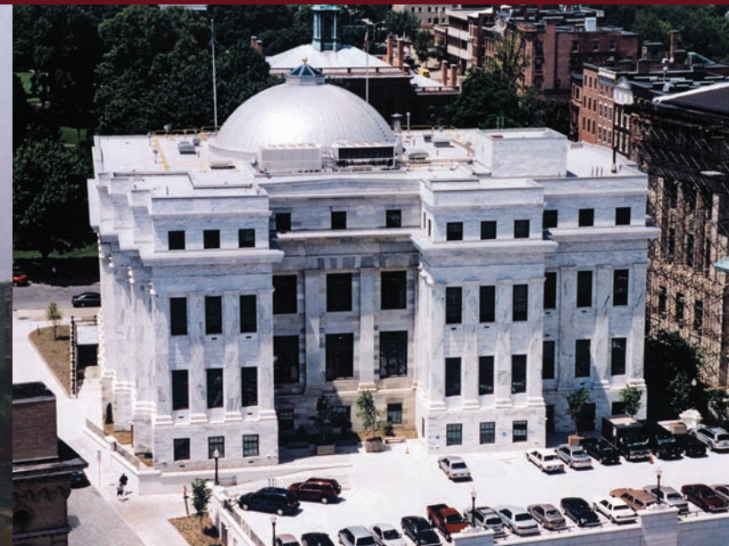
Rear view of Court of Appeals Hall after the 2004 renovations
