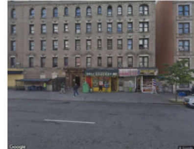
1516 AMSTERDAM AVENUE, MANHATTAN currently has 114 open HPD violations - the most in this portfolio.
