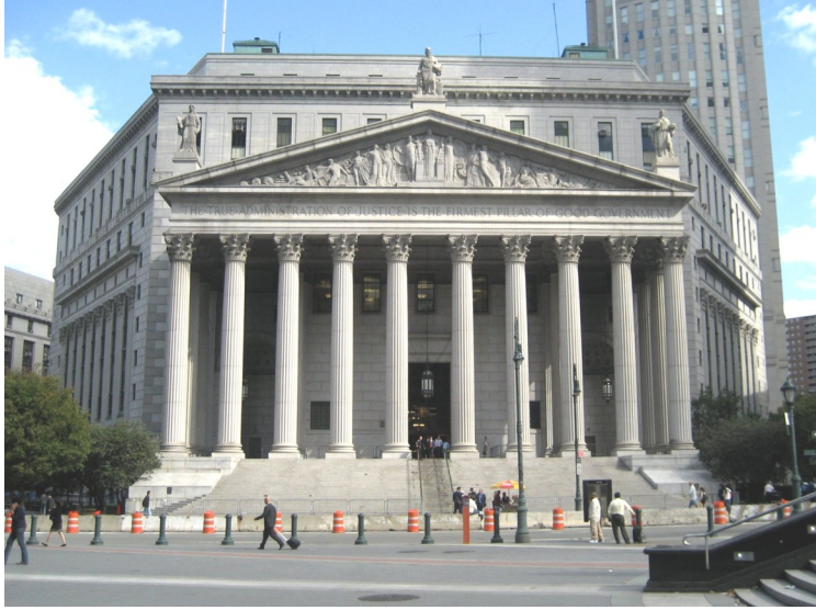
Portico and main entrance
